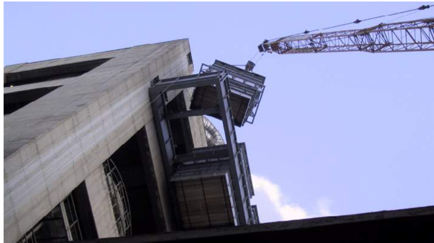
STRUCTURAL REINFORCEMENT OF A PRE-HEATER TOWER
