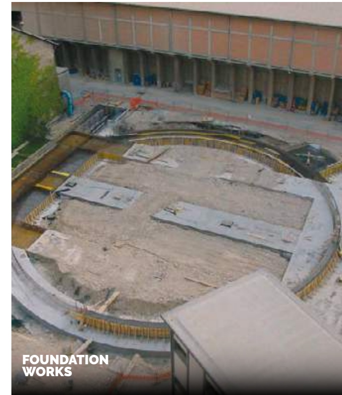
REALISATION OF A CLINKER SILO IN REINFORCED CONCRETE
